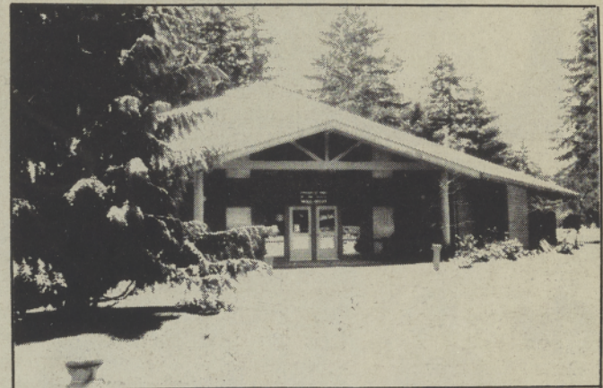
A blanket of snow covered the Siletz Area Central Office and most of Western Oregon
