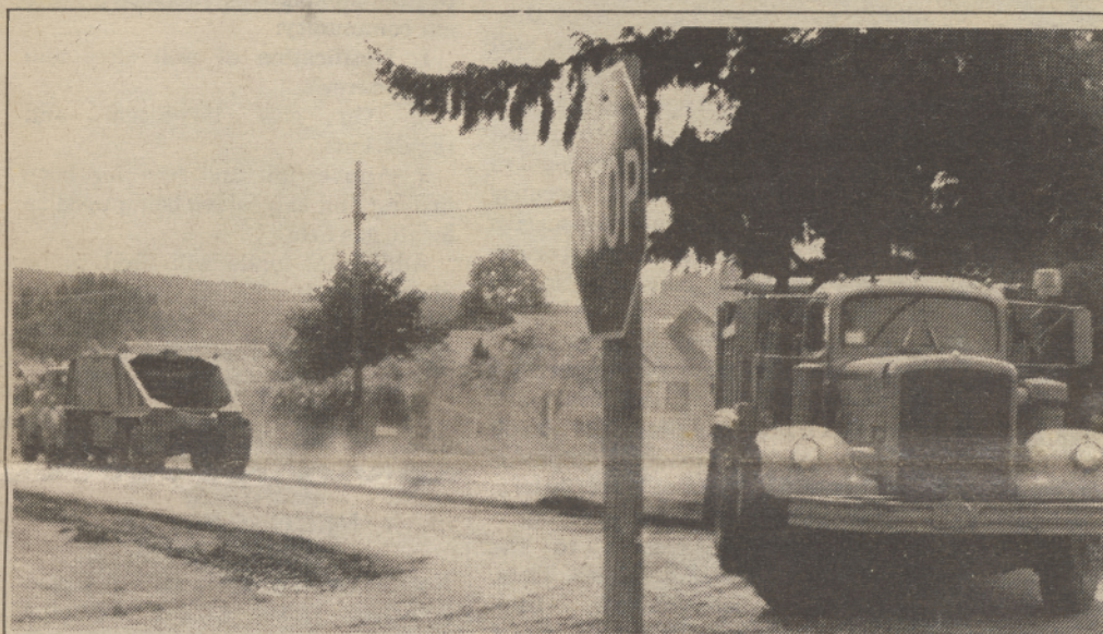
ROAD WORK— As promised by the State Highway Department, Bridge St. from the Nehalem River Bridge to the Fire Hall, is being widened by six feet. The job is expected to reach completion near June 1.
