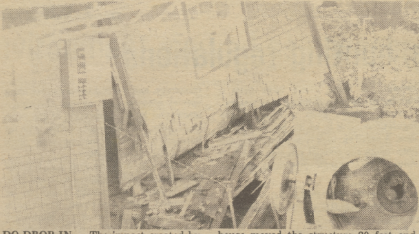
DO DROP IN — The impact created by Joe Banzer's car as it crashed into this house moved the structure 20 feet and split the building in two. FREEDOMFOTO
