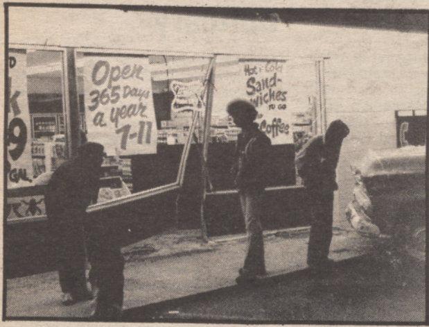
Accident occurred last Tuesday, with pick-up truck driving into the Mini-Mart for drive in delivery. Unfortunately window was in the way.
