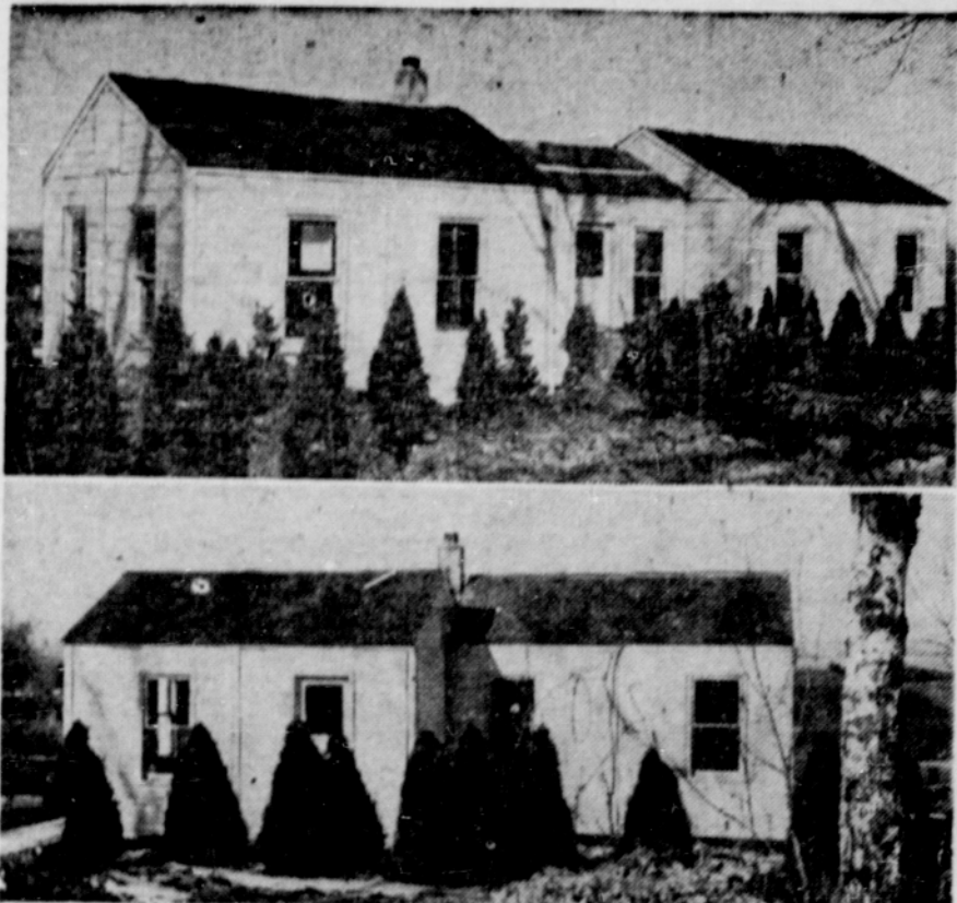
GRAIN BINS ARE HOUSES . . . The Shenandoah (Iowa) chamber of commerce is doing something about the housing shortage. Above are two houses made from surplus grain bins. The top house has three rooms, all shown. The lower house has a utility room in the rear which cannot be seen. Both have bathrooms, two bedrooms, living room and kitchen. The original grain bins were 14 by 16 feet.
