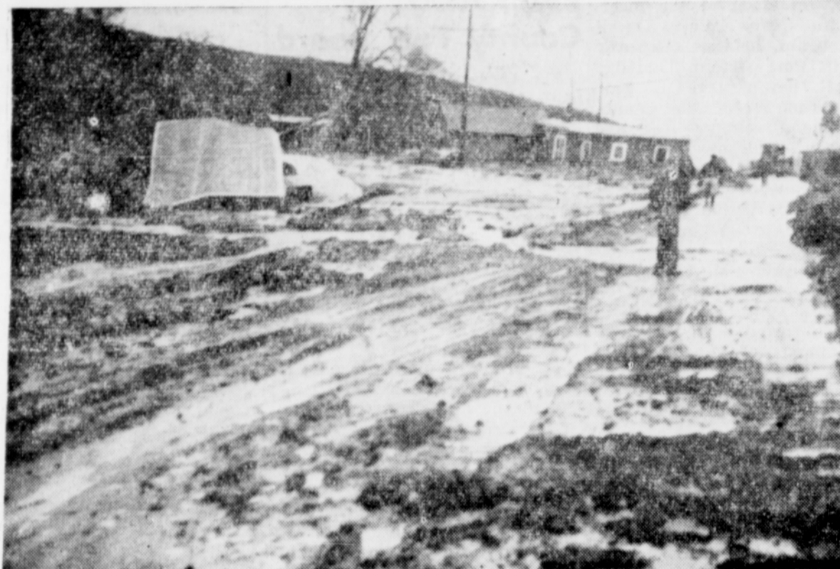
THE HENRY LABARGE home (background) and garage (foreground) that slid onto Highway 101 during the recent storm. This picture also shows somewhat the condition of the highway.
