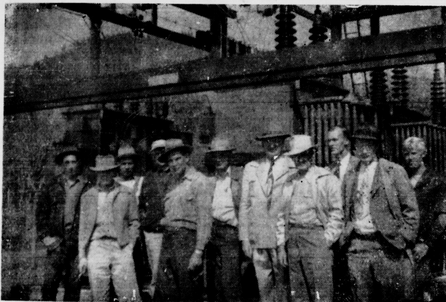
View of new transformer at Gold Beach, where electricity was turned on last Monday, at completion of $350,000 REA transmission line from Brookings.
