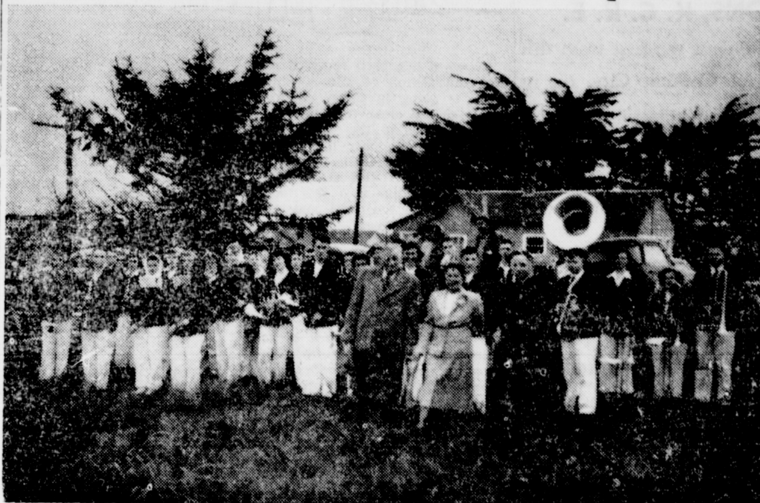
Breaking ground for the new Curry County Hospital at Gold Beach. Dr. W. A. Cartwright, mayor, Mrs. George Mateer, who worked tirelessly on the project, Rev. Sydney Walker, D. D., and G. C. Humphreys with the Gold Beach high school band. Story on page two.
