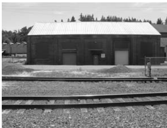
7TH STREET MOUNTAIN STATES POWER STATION 1997 (ABOVE) AND IN 2002 (BELOW)
