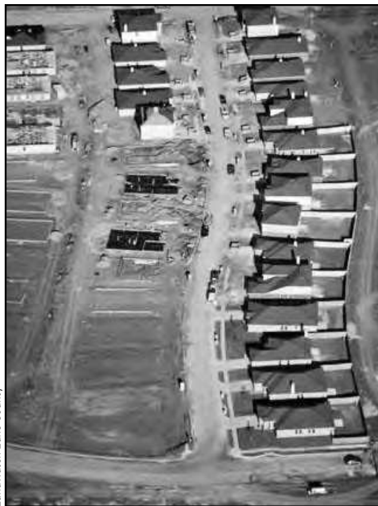
LandWatch Lane County
