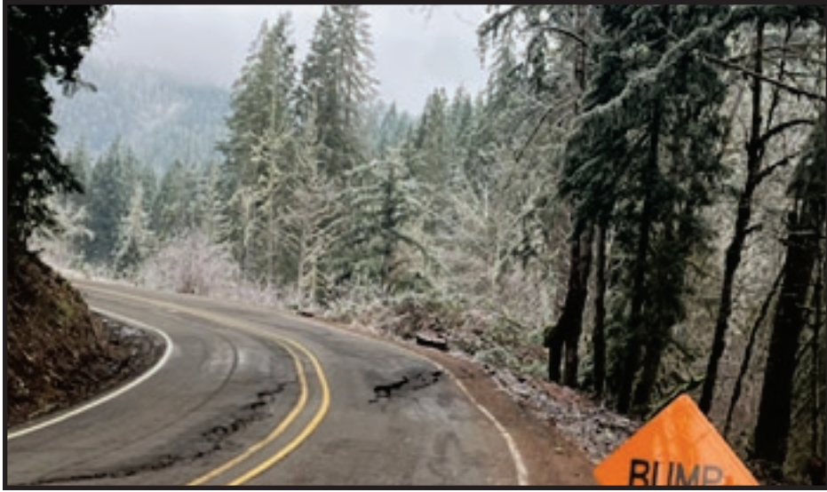
Above In North Douglas county out on Smithville Rd. Freezing water has played havoc on this county road. Asphalt is cracked open. Photos by Russ and Charlotte
