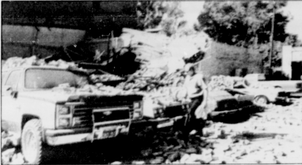
PASADENA, CA — This single story building built in the early 1900s crumbled to the ground during Southern California's earthquake which measured 6.1 on the Richter scale.
