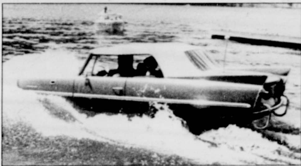
BEND, OR — A 1965 Amphicar drives into a lake. Two propellers extend from the car's rear and the front wheels act as rudders. Only 3,000 cars were made.
