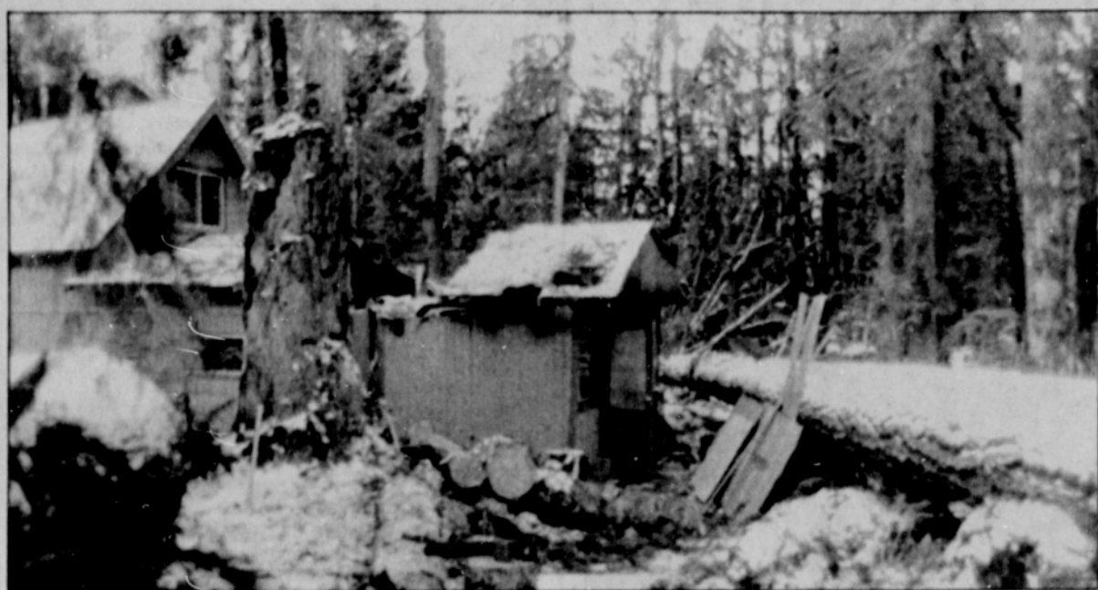
Damage was extensive to the Bill Ellis home.
