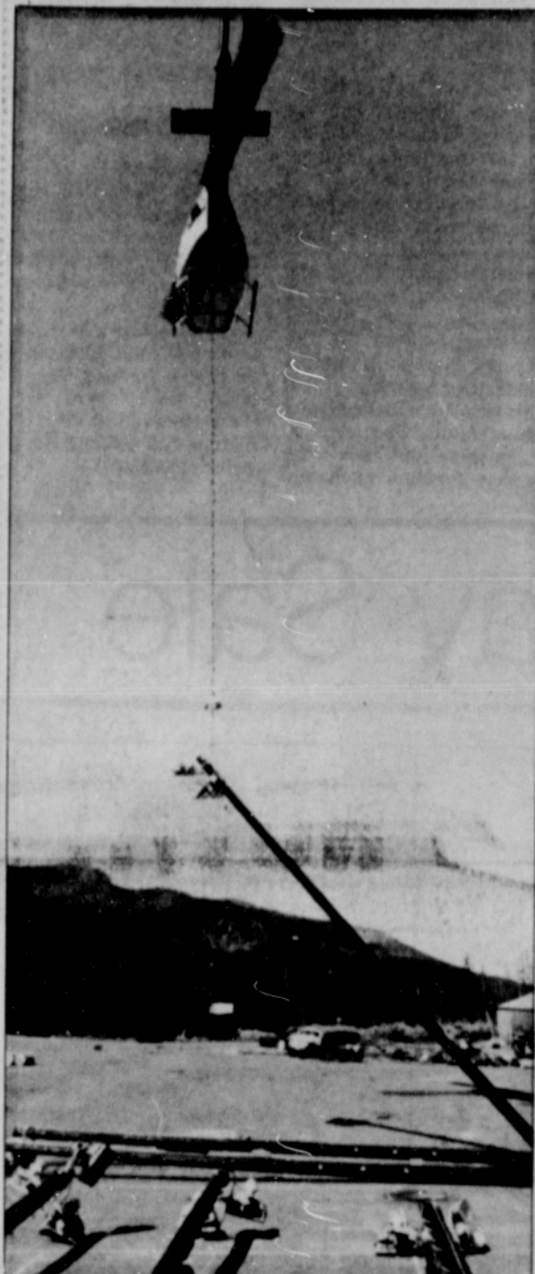
Helicopter installs new light poles at Multorpor.
