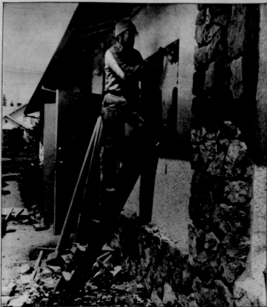
Staff photo Volunteer contractor Chuck Spradling of Mt. Hood Hospice puts in windows in new Hospice quarters in the Sandy Post building at 17270 SE Bluff Road. The group that offers free home care for terminally ill recently moved from Heritage Square to the former site of Sandy Printing and plans a June 10 open house in conjunction with The Post.
