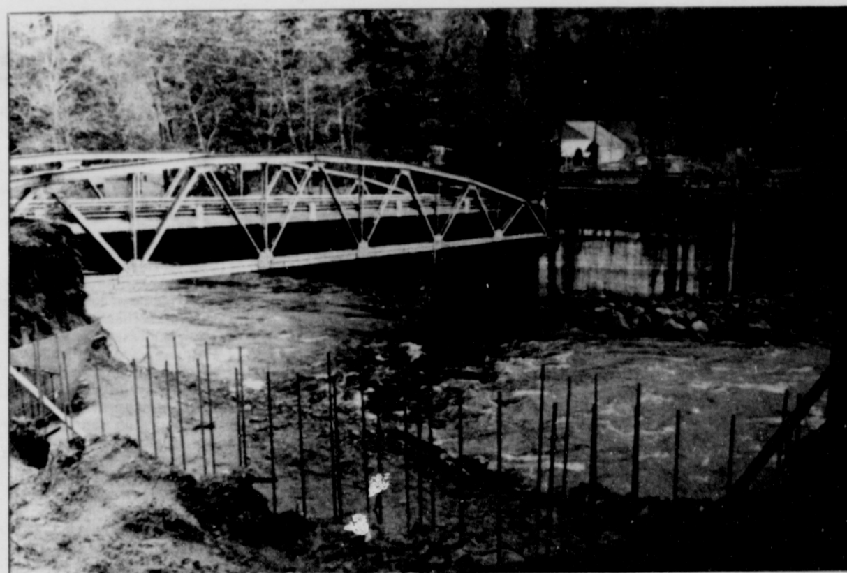
Foundations have been poured as work is underway to renovate and widen Sleepy Hollow Bridge.
