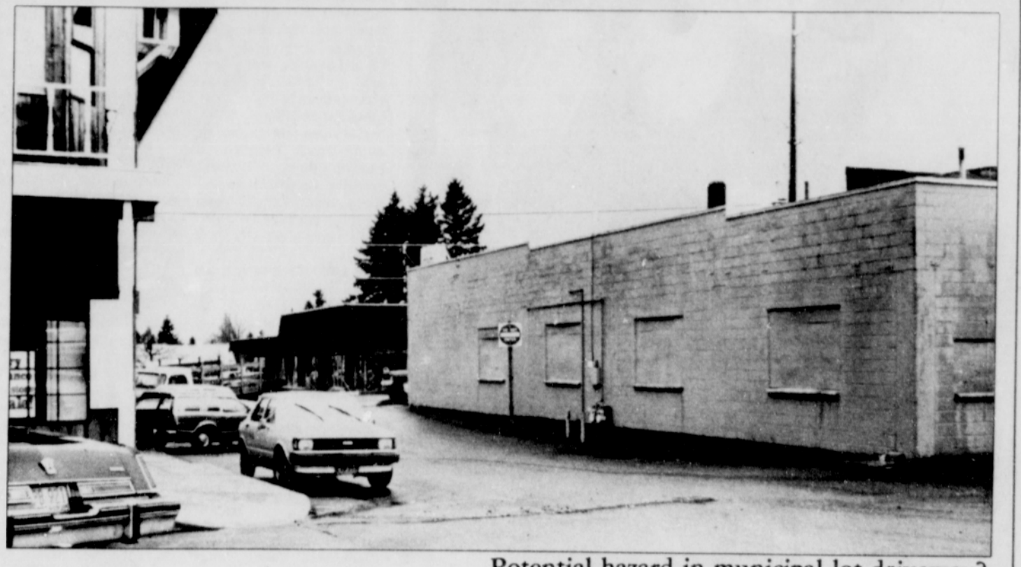
Potential hazard in municipal lot driveway?
