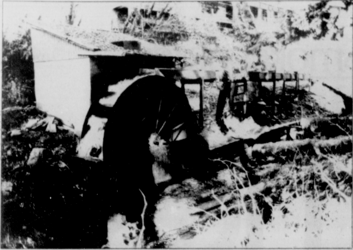
Cal Horger's water wheel has become one of the most efficient sources of alternative electricity generation in the Portland General Electric Co.'s customer area. Staff photo
