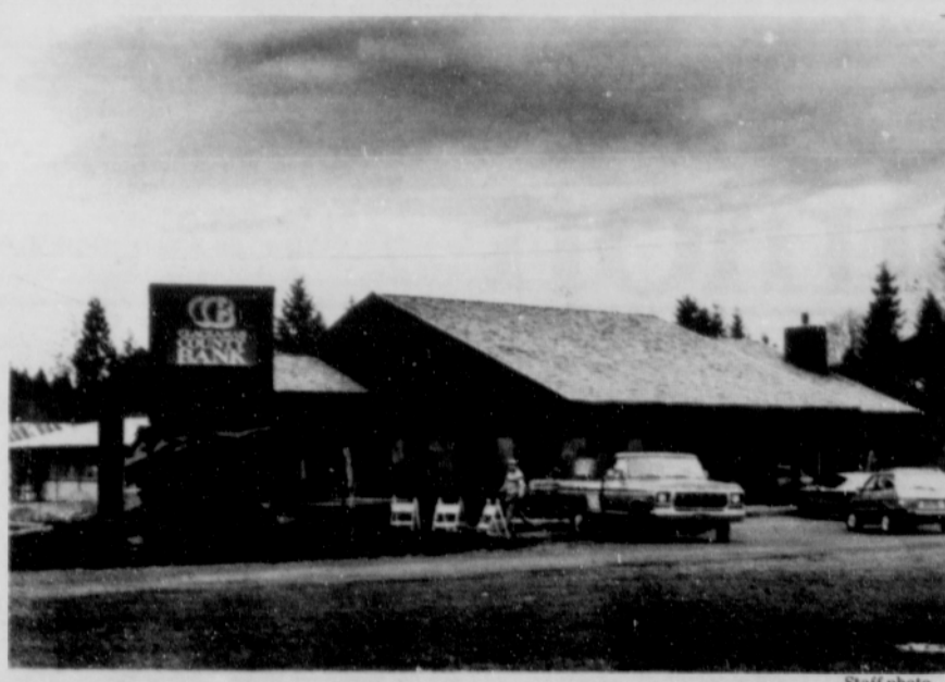
The remodeled Hoodland branch of Clackamas County Bank will be featured in an open house next Thursday.
