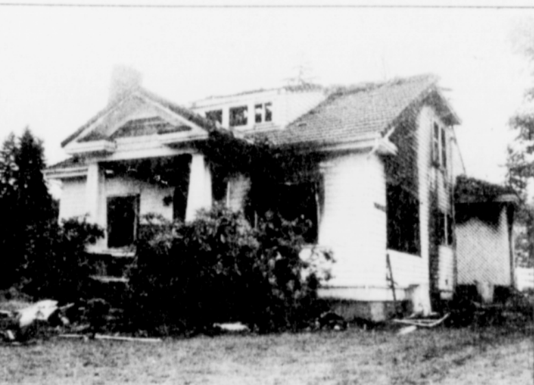
Fire was blazing from the front windows of the home when firefighters arrived.
