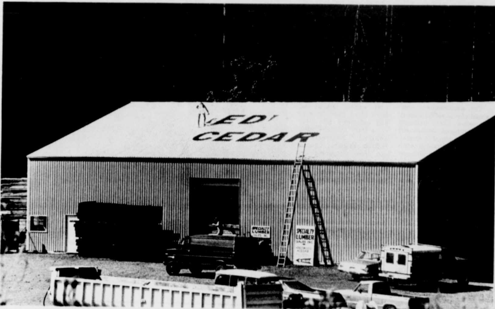
A workman at Specialty Lumber Sales, Inc., painted over the building's roof sign Tuesday. City ordinances don't allow such signs, however, city officials have worked with owners of Mt. Hood Industrial Park to provide a new sign
