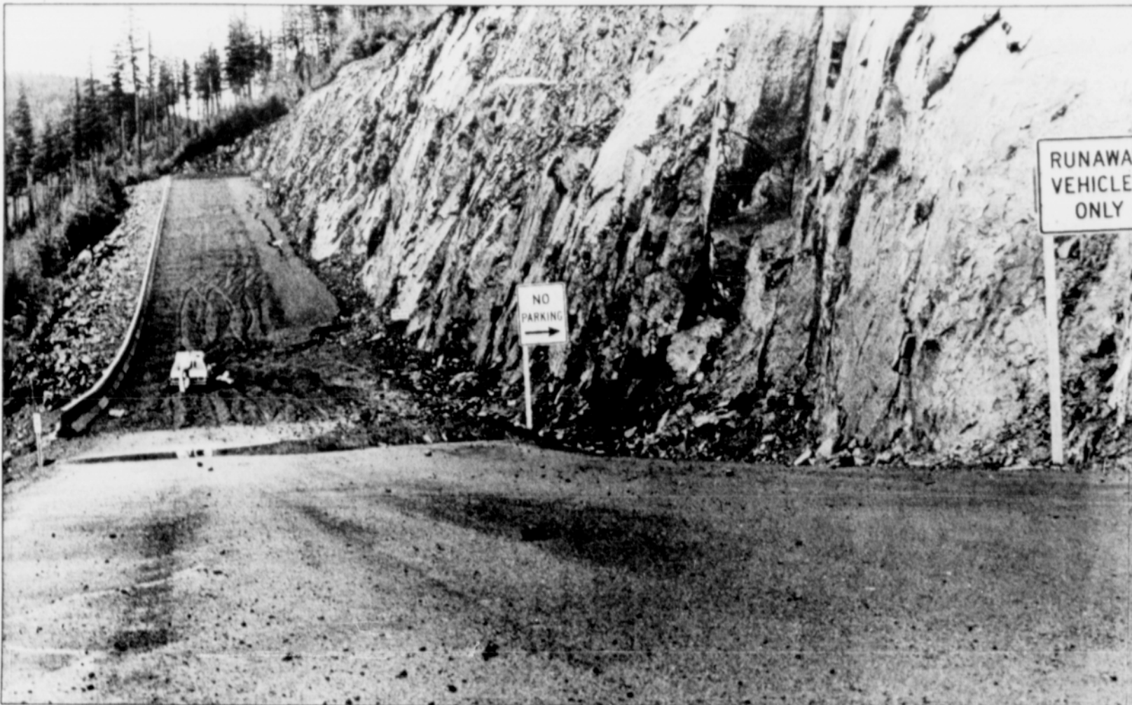
The runaway vehicle ramp on U.S. Highway 26 continues to provide mountain traffic with a safety outlet for speeding vehicles. This car used the
