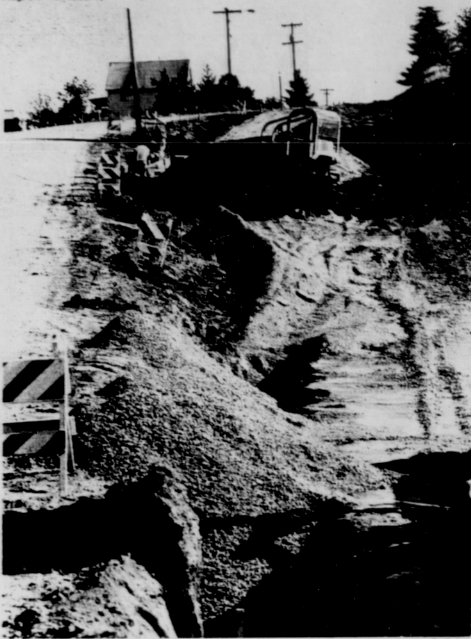
Work is underway to straighten South Bluff Road. Monday night the city council OK'd a plan to put a base under the asphalt from Nettie Connett to Sandy Heights Street. The country road had no such base placed when it was made. It will cost an additional $5,000.
