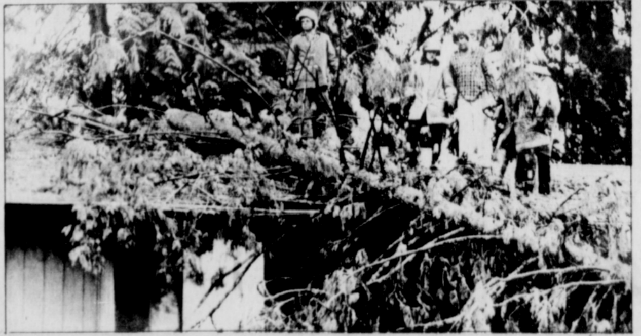
The Barry Fretz family had just finished dinner when this tree crashed through the roof right above their
