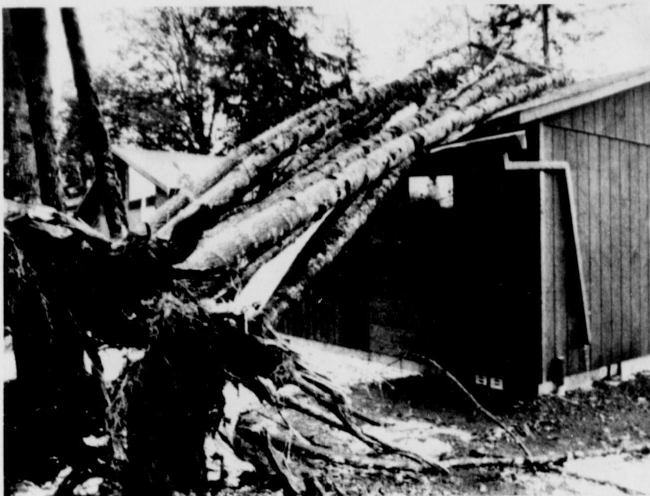
High winds Monday evening uprooted trees and sent them crashing into the roofs of two homes in the Aldergate
