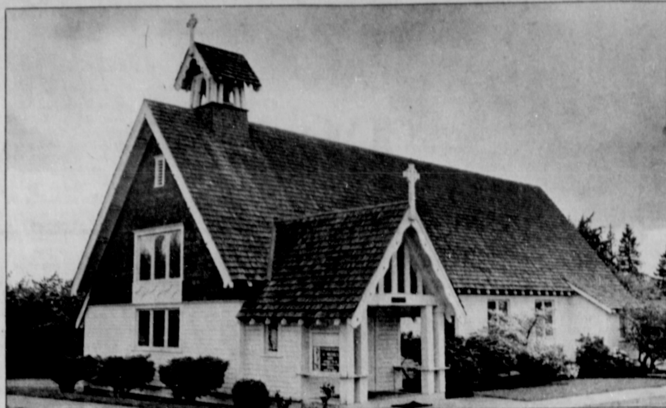
ST. MICHAEL'S Catholic Church will move to a new home soon. The congregation will move from its Strauss Street location to a new church on Langensand Road, if the City Council approves.
