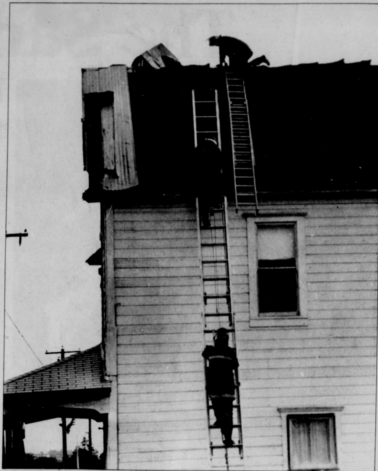
Roof flies apart in wind
