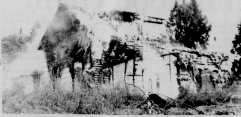
CLEARING LAND for Henderson-McNeely's new 84-home Tickle Creek Estates subdivision behind Sandy's Industrial Park on Southeast 362nd
