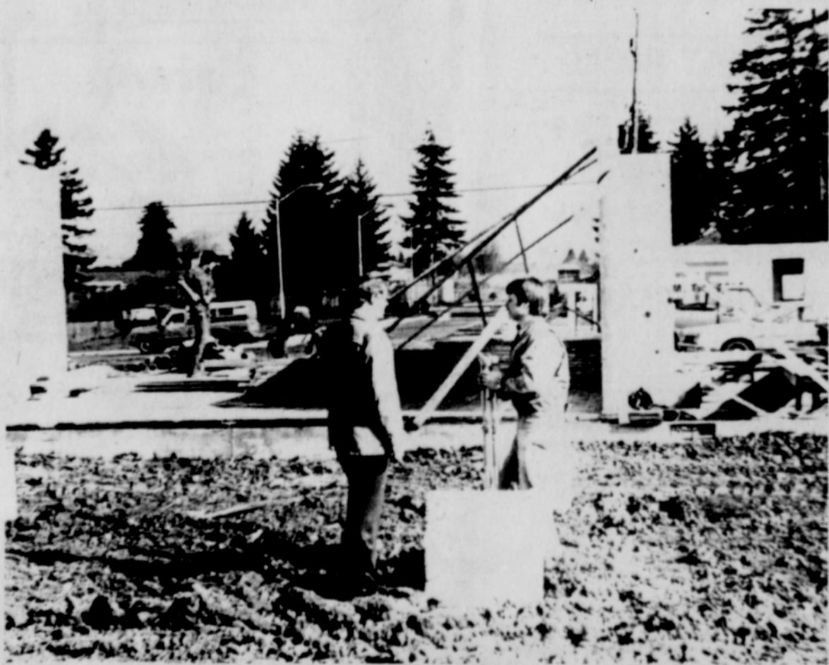
- Building the new Clackamas County Bank
