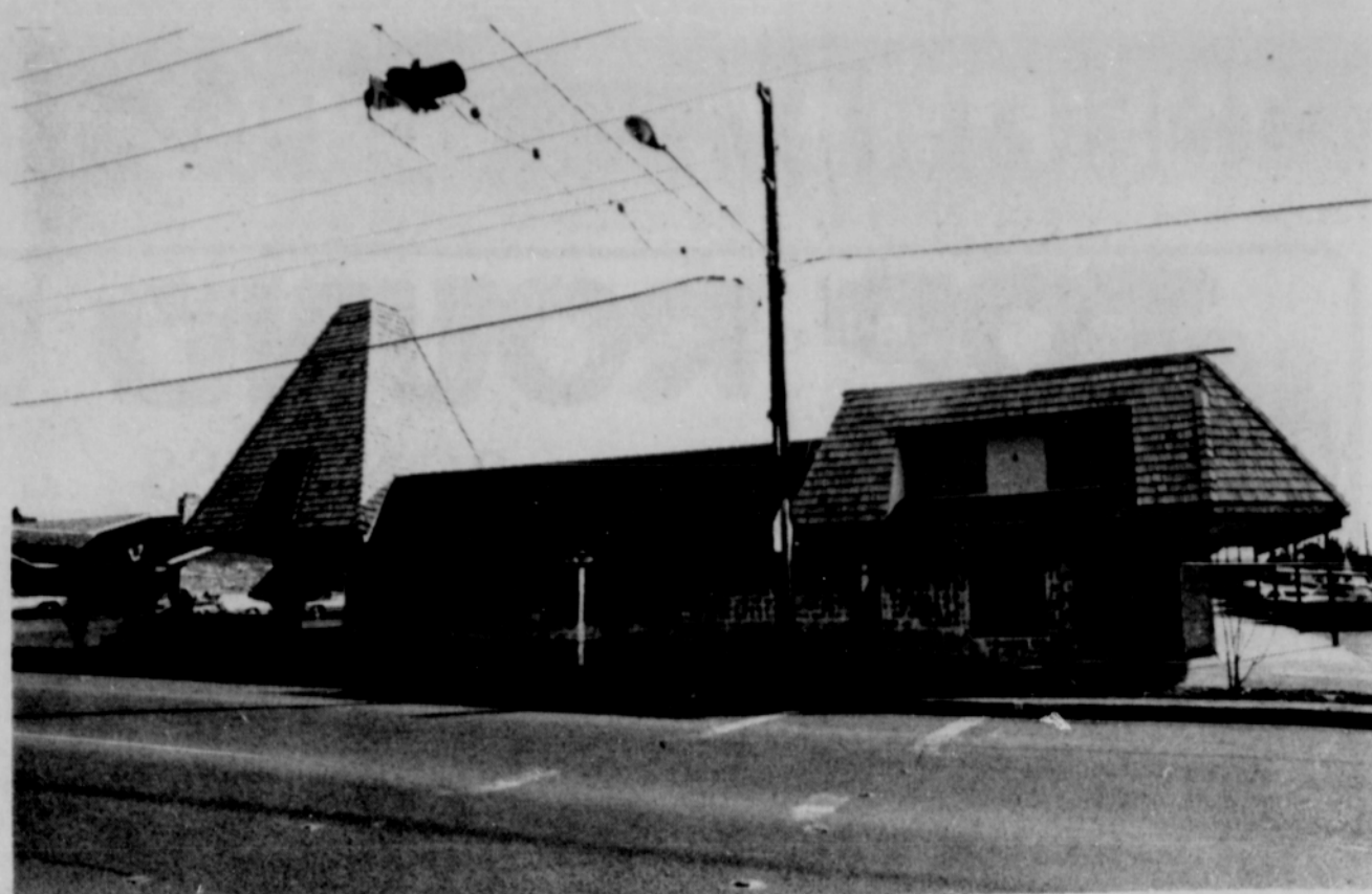
Gordon Stone Building
