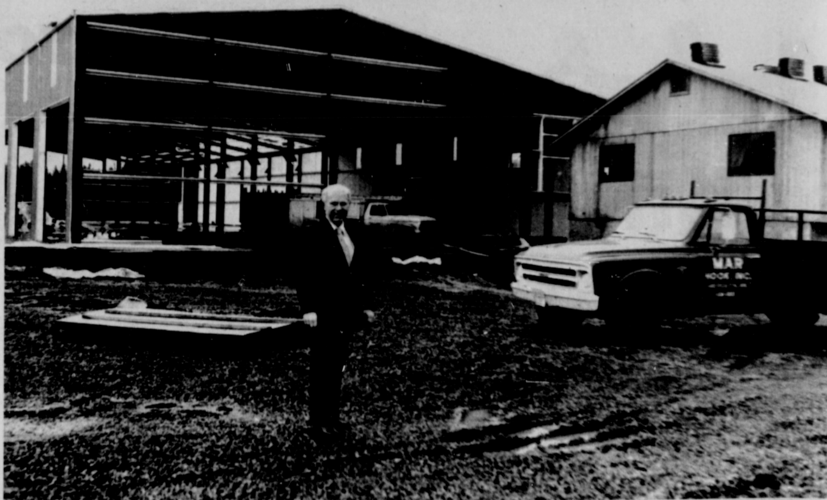
JOHN MITCHELL, president of Mar Hook Company, has been making regular trips from Aberdeen, Wash., to see progress on the company's new plant in the Sandy Industrial Park.
