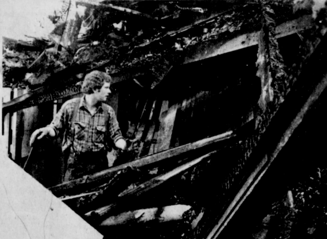
MAINTENANCE SUPERVISOR Larry Gusinger of the Son Village assesses the damage.
