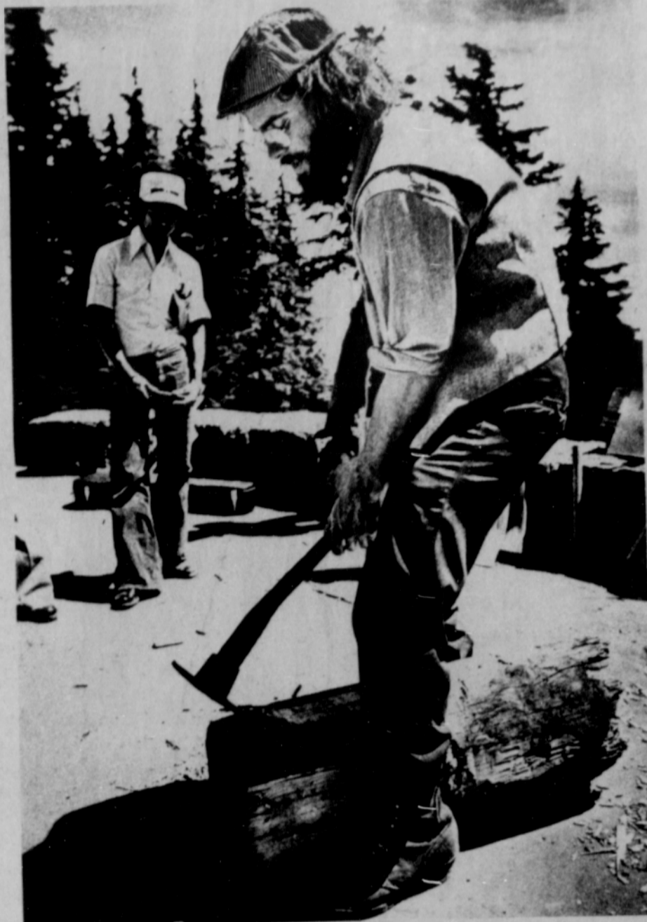
JEFF POST demonstrates the methods used to build Timberline Lodge.
