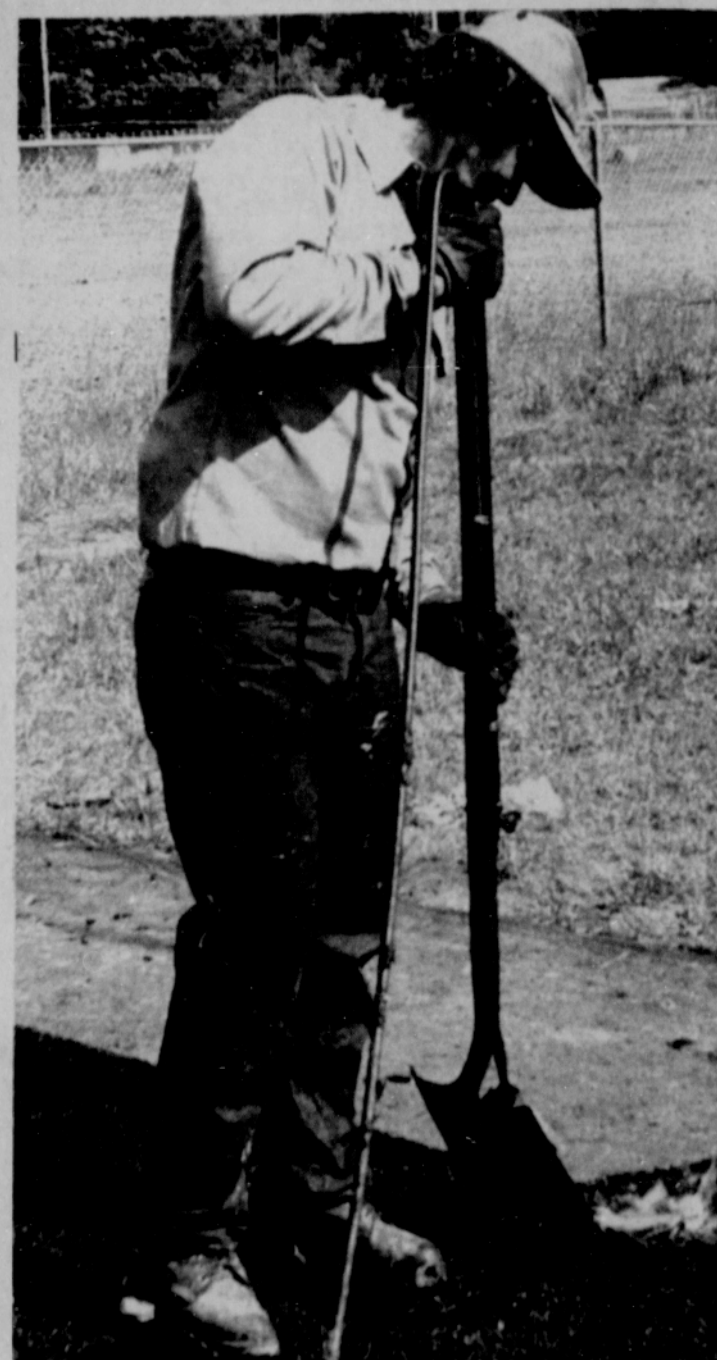
PHASE III of the building program at Sandy Union High School recently began and construction worker did some black topping at the entrance to Stadium last week. Construction work will continue throughout the summer on the high school physical plant.
