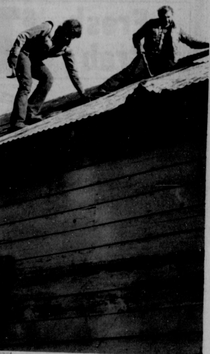
TED GARLOCK, left, and Don Predmore are working this week on demolishing the old Berry and Son building on Pioneer Boulevard. The two will use wood salvaged from the building for construction of barns.
