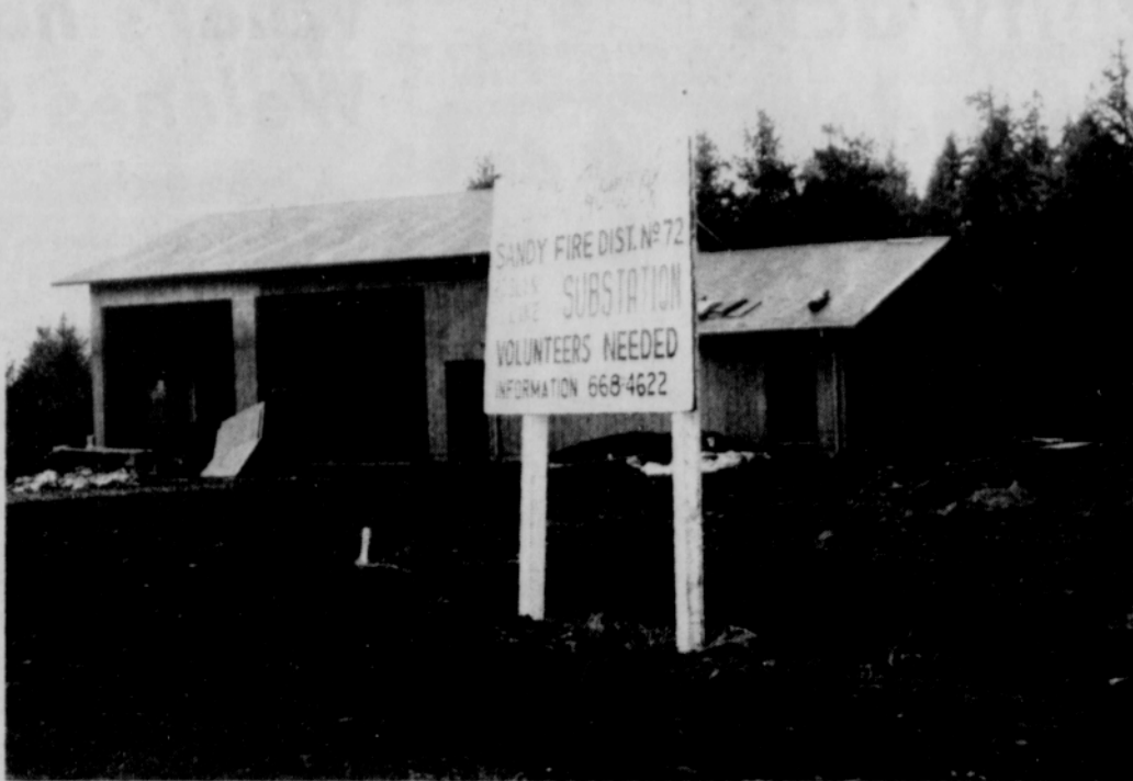
SANDY FIRE District No. 72's newest substation is almost ready for occupation and operation. The new structure is located in the Roslyn Lake area. (Post Photo)
