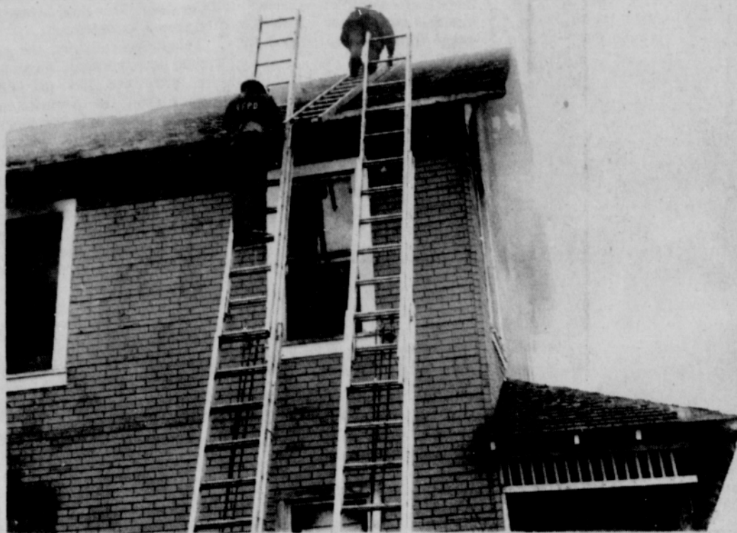
THE PROPER use of ladders and instruction on cutting a hole in the roof of a house for ventilation purposes were two of the subjects which were taught at last
