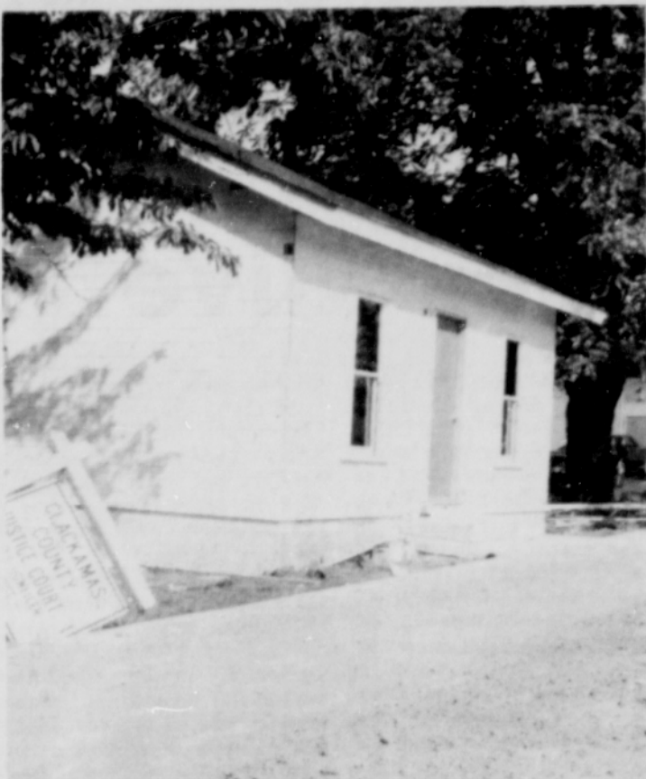
REMODELING WORK is about completed at the offices of Howeler and Richards. The new addition has given the building a new look. This work was cited for helping improve the look of Sandy by the local chamber. (Post Photo)
