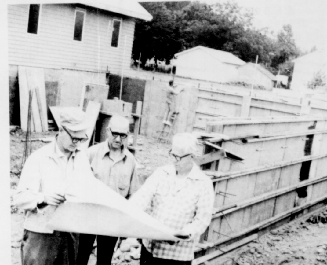
ROSE OF SHARON Lutheran Bretheran Church building expansion was well under way this week. Julius Johnson, left, John Paulson and Pastor Otto W. Brustad, right, check out plans for the new sanctuary-Sunday school addition. Kent Construction Co. is doing excavation and concrete work. The congregation will finish the remainder
