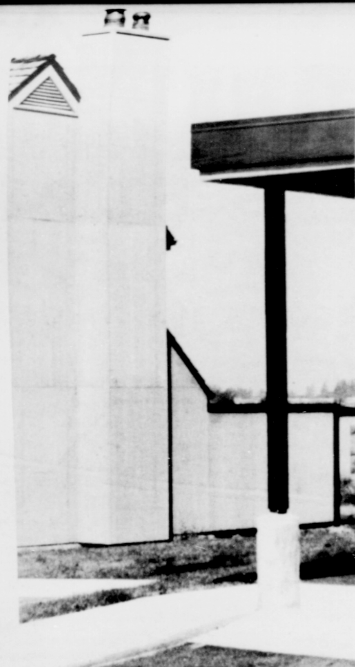
CHIMNEYS GO to pot in new development called Bull Run, north of SE 1st. Each structure sprouting chimneys has diversity from the others.
