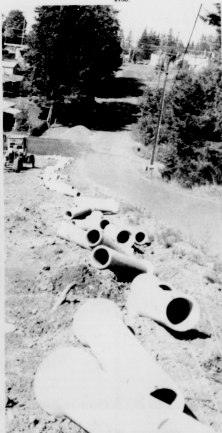
THE CITY has begun work this week to extend the sewer system to the Sandy Heights area. Here sewer pipe is awaiting work crews along S. Bluff Rd. (Post photo)
