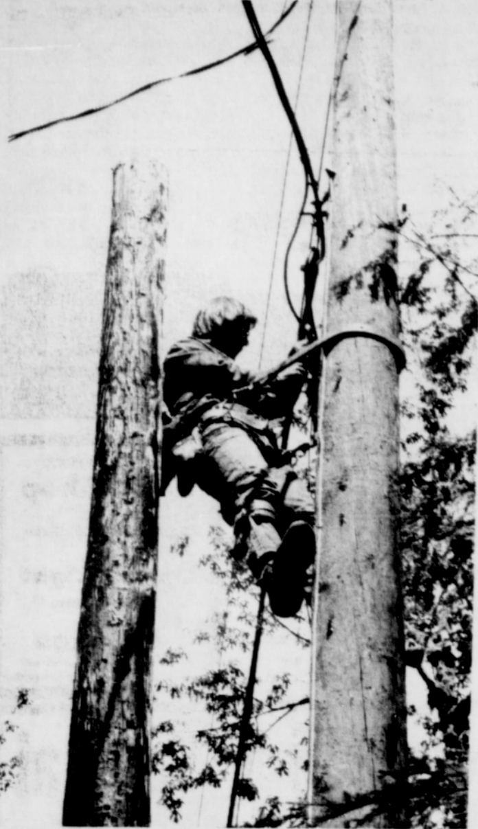
JERRY BEACH, technician for CableVision in the Hoodland area, installs new equipment which will help better service in the Aldercreek, Lolo Pass and upper Rhododendron areas, according to a company spokesman. The mountain television cable system is currently working on an expansion program.
