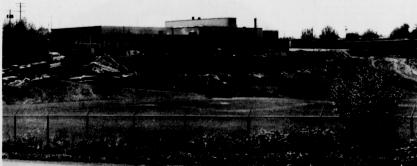
AUG. 15 is the completion date still planned for the new upper grade wing at Sandy Grade School. The wing will house upper grade rooms and vocational classrooms. It is a two story building. The
