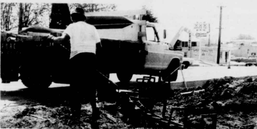
CREWS ARE now working on the corner curbs along Proctor Ave. Here a workman works on the corner of 3rd Ave. and
