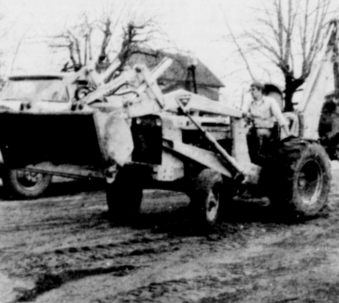
OLD BACKHOE is used in conjunction with new one to save time in digging operations now in progress on Proctor Avenue. (Post Photo)
