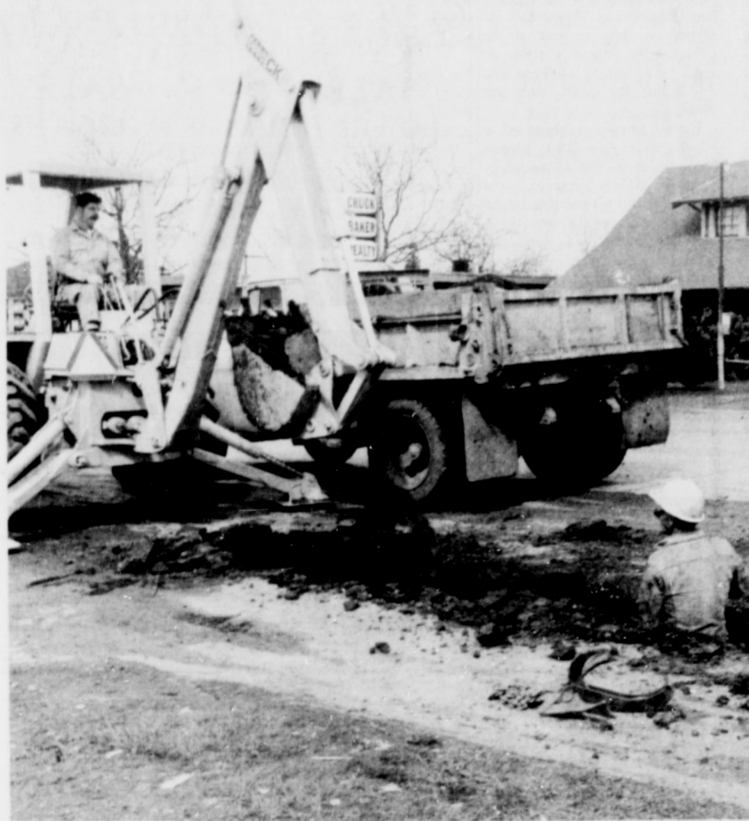
KEN BURDICK, public works superintendent, tries out the new backhoe recently purchased by the city. Ditch is on Proctor
