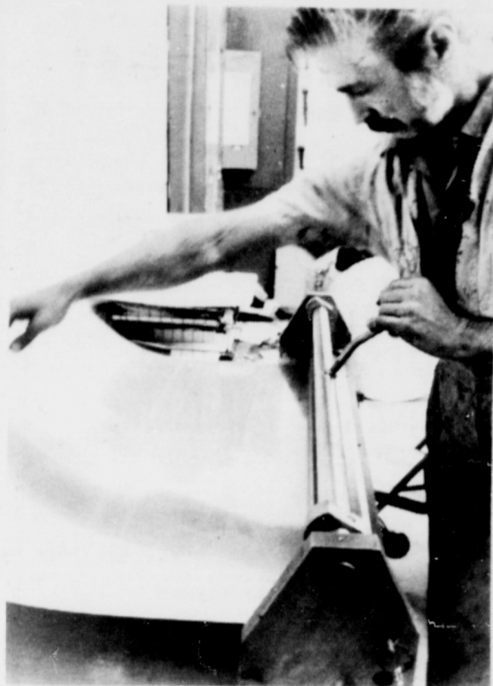
ON A BENDER. Ed White, press foreman, puts a crimp in plate so it can be secured in printing cylinder. (Outlook photo)
