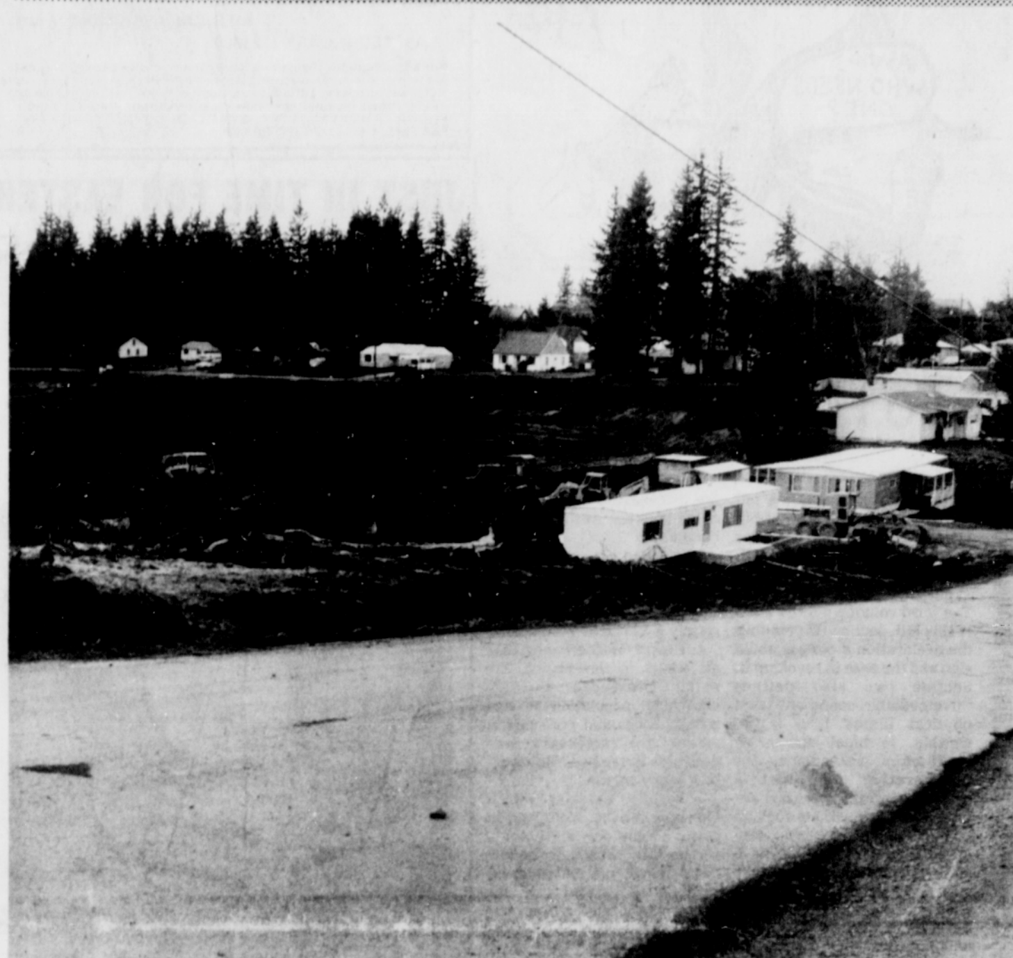
THIS PHOTO shows how the land has been stripped for the development of a trailer park in Sandy. The park will be located off of S. Bluff Rd. and Sunset St. Already two trailers have been moved into location along S. Bluff. While the work for the trailer park is being done, the city is having the work done to straighten S. Bluff Rd. (Post Photo)
