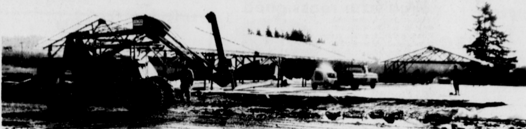
DAMASCUS THRIFTWAY Shopping Center is under construction at Damascus for Damascus Development Co.
